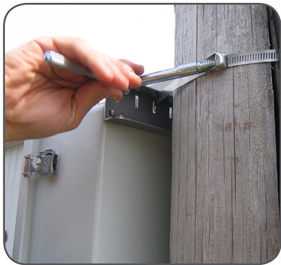
Pole mount brackets secured with wire and screw clamp
