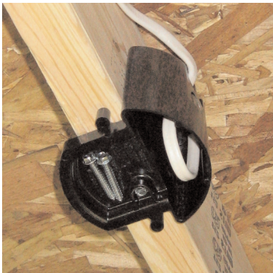
9375-FR shown mounted on a ceiling joist prior to mounting a paddle fan
