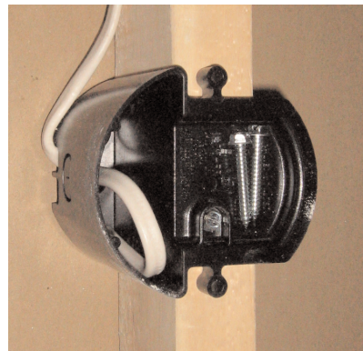
9375-FR shown mounted on a wall stud prior to mounting a light fixture
